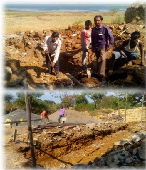
Construction of Grave Yard at Nagosali Village
